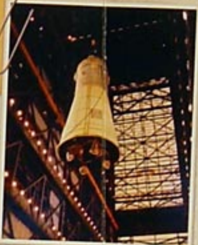
The Apollo spacecraft is hoisted up to be lowered into the top of the Saturn V rocket. At the bottom you can see the footpads of the Lunar Module inside the craft.
