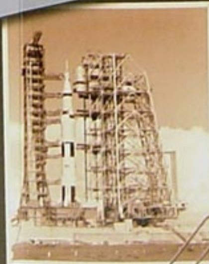
The Apollo 11/Saturn V begins its roll-out from the VAB to Launch Complex 37-A, which is where it will take flight. The Crawler-Transporter operates using caterpillar tracks to move the stack.
