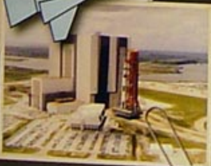
The Apollo 11/Saturn V begins its roll-out from the VAB to Launch Complex 37-A, which is where it will take flight. The Crawler-Transporter operates using caterpillar tracks to move the stack.
